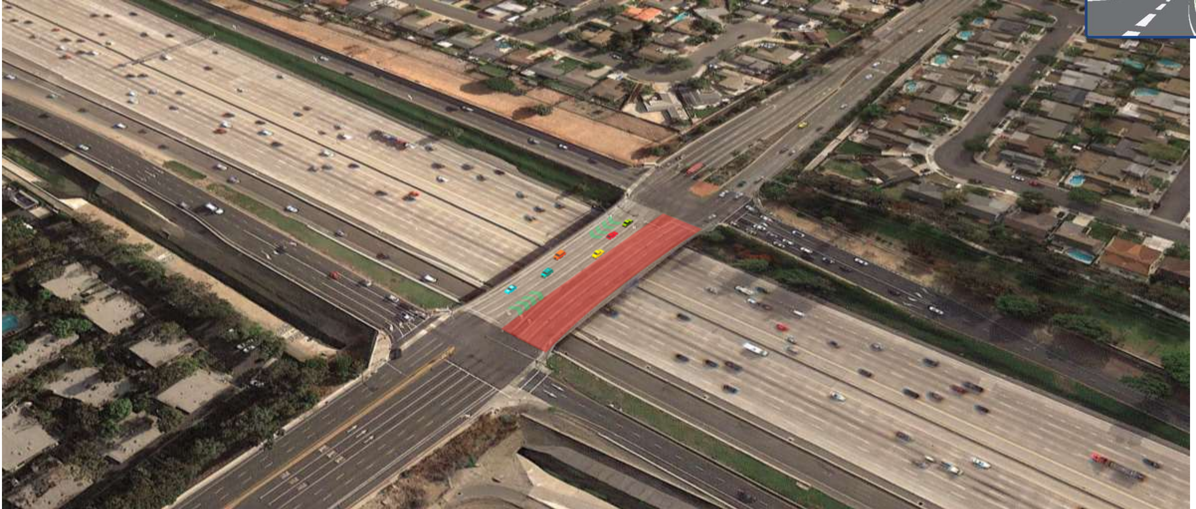
Traffic Moved to East Side of Bridge
