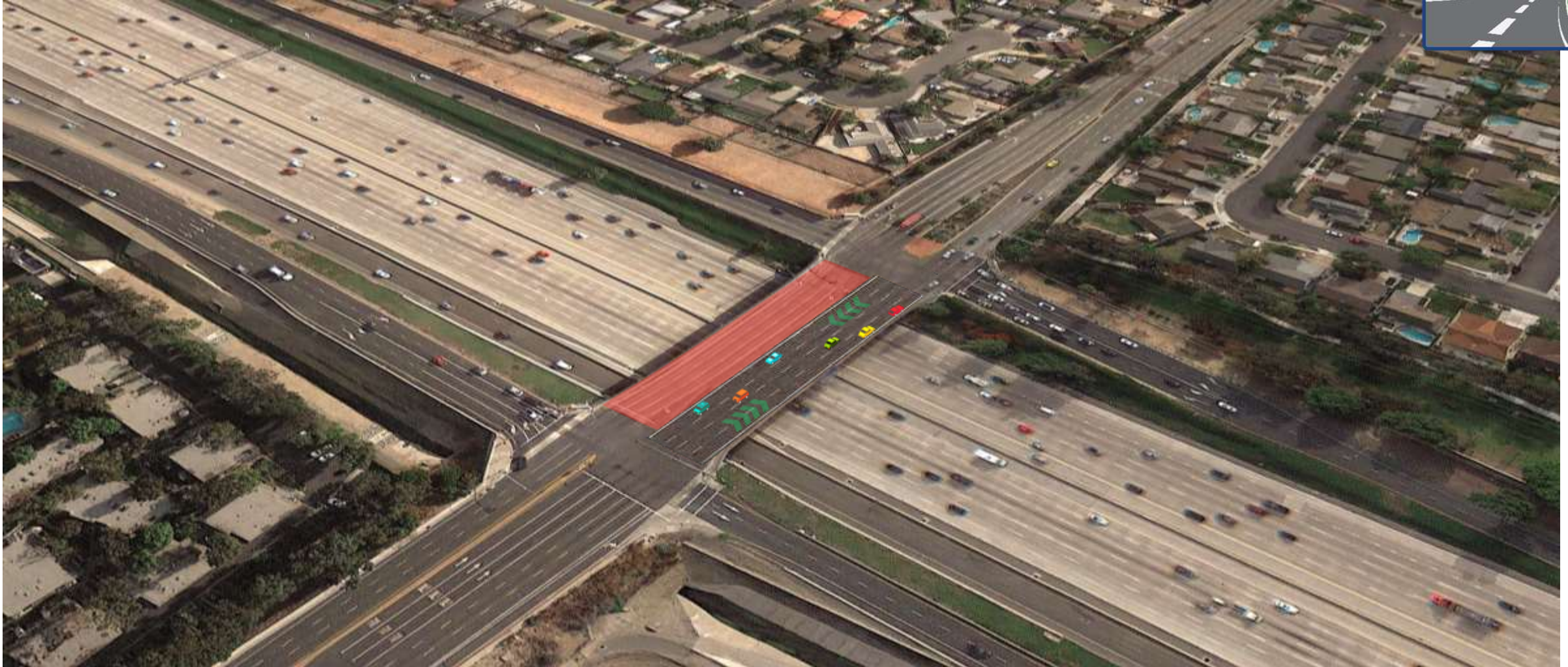
Traffic Moved to West Side of Bridge
