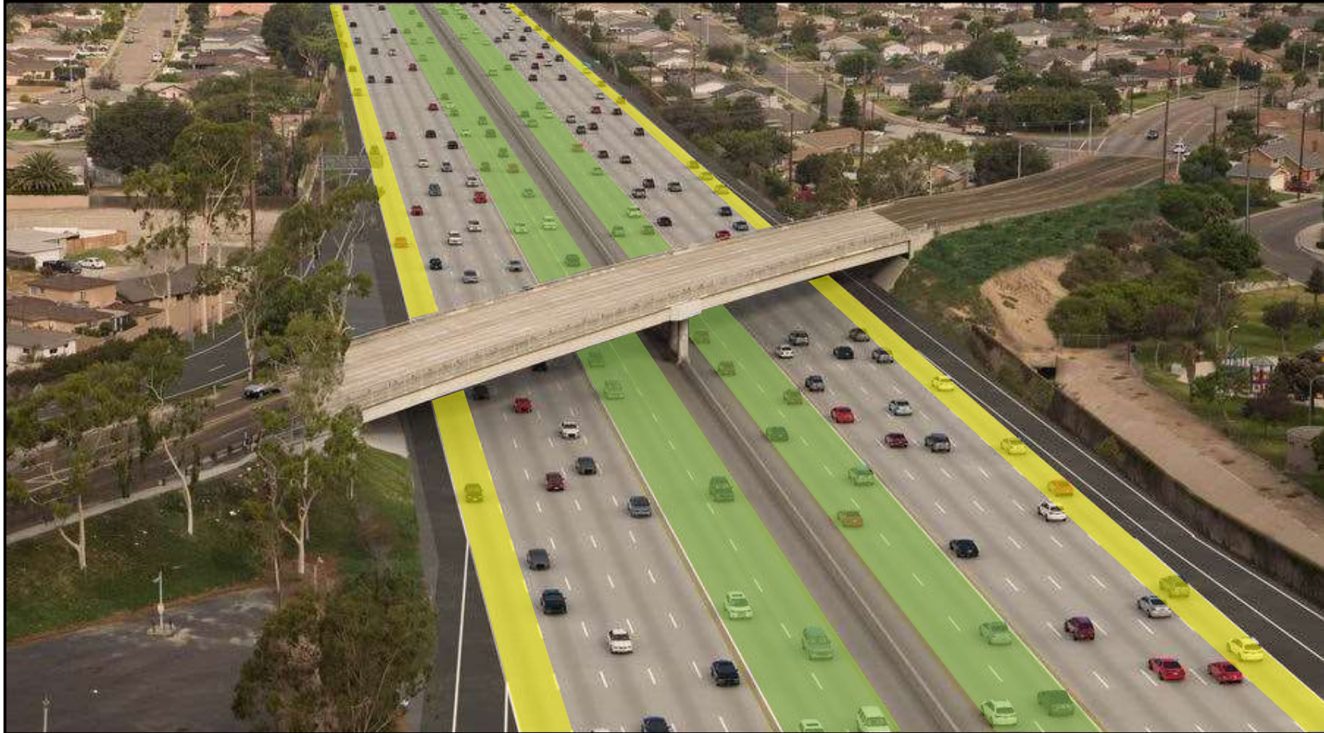
I-405 looking northwest at Springdale Street bridge
