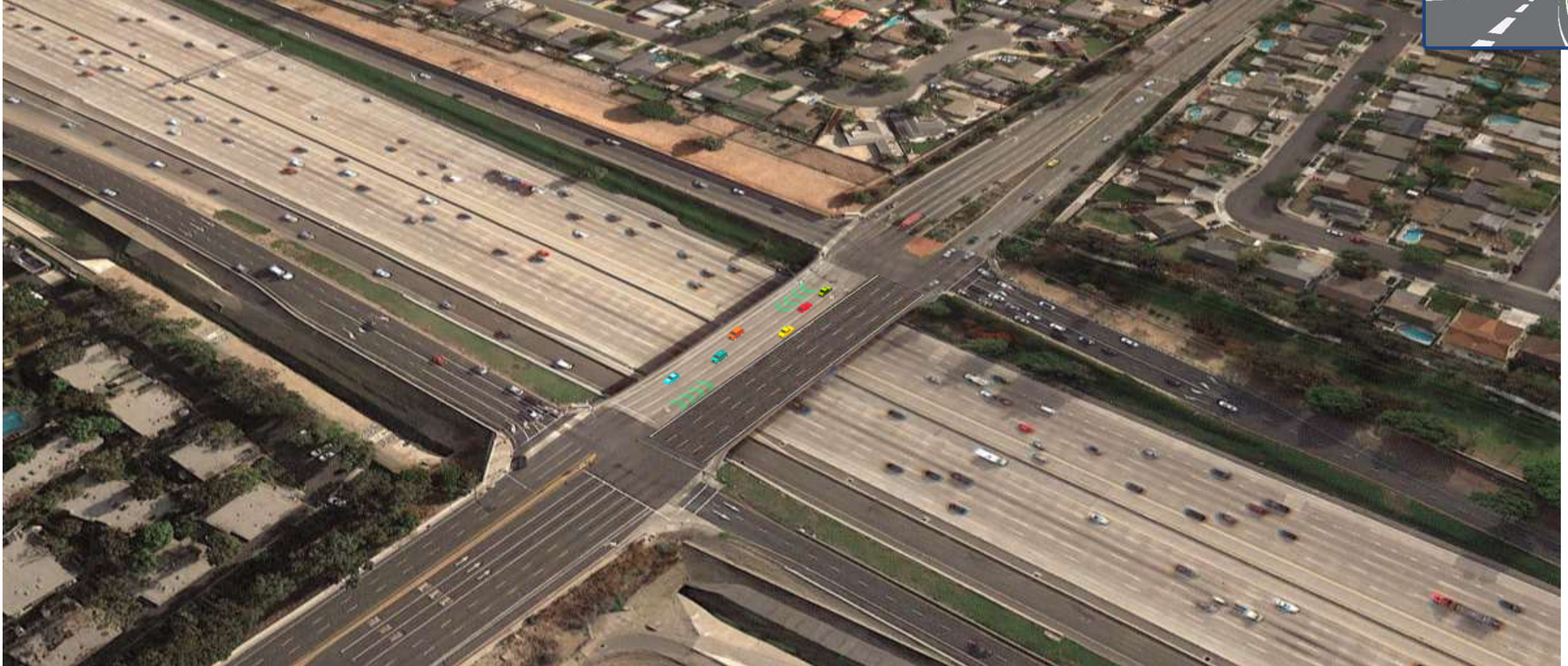
West Side of Bridge Replaced
